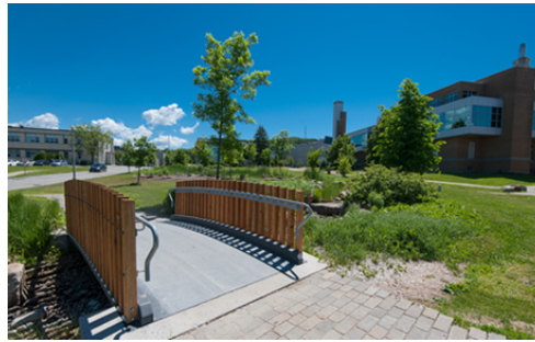
Figure 2. UHPGC Footbridge built at the University of Sherbrooke.
