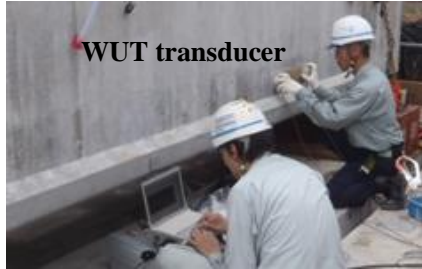
Figure 1. Grout inspection using the WUT.
