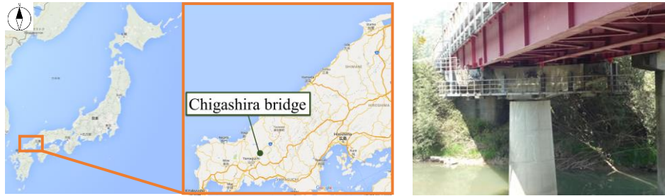
Figure 1. Location of Chigashira Bridge.
