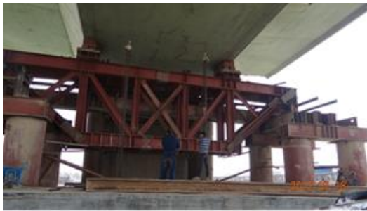
Figure 5. Reinstating original structure.
