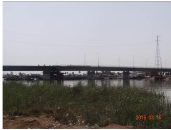
Figure 8. Bridge after connecting both structures.
