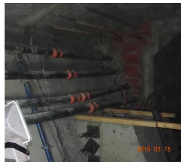
Figure 4. Inside end of new structure.
