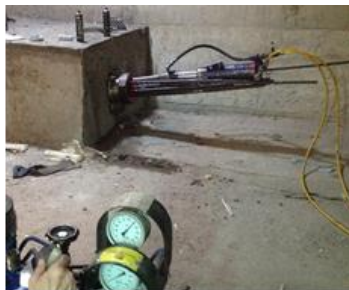
Figure 7. Anchoring old tendons.
