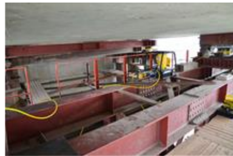
Figure 6. Reinstating original structure.
