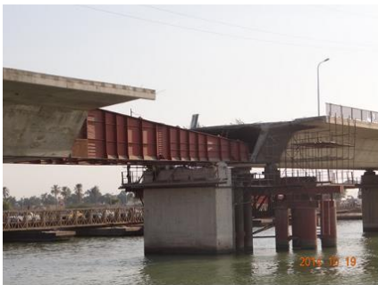
Figure 3. New spans and launching nose.
