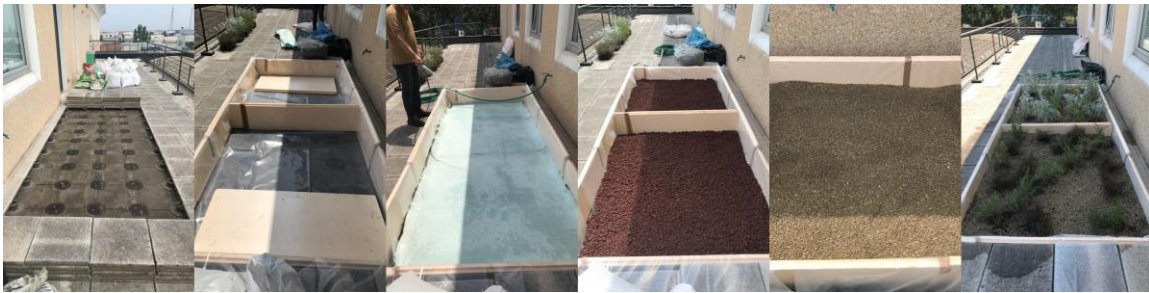
Figure 2. View of the main phases of the green roof implementation.
