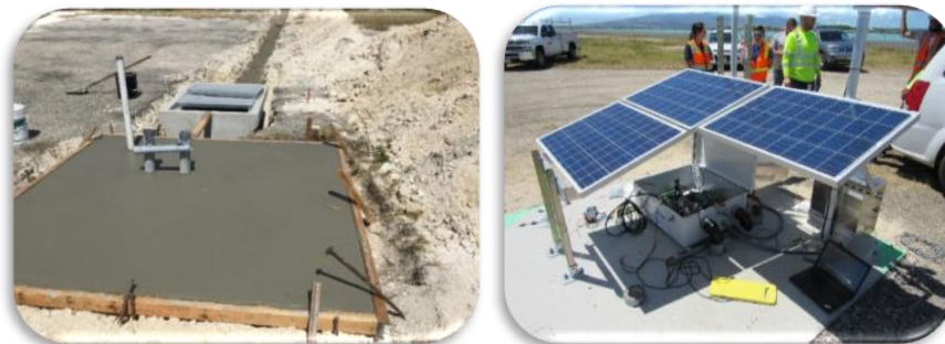
Figure 5. DAQ platform concrete and equipment.
