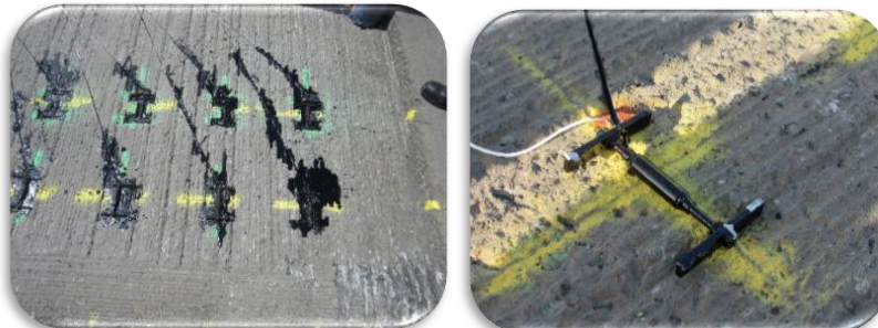
Figure 4. Sensors are secured in place.
