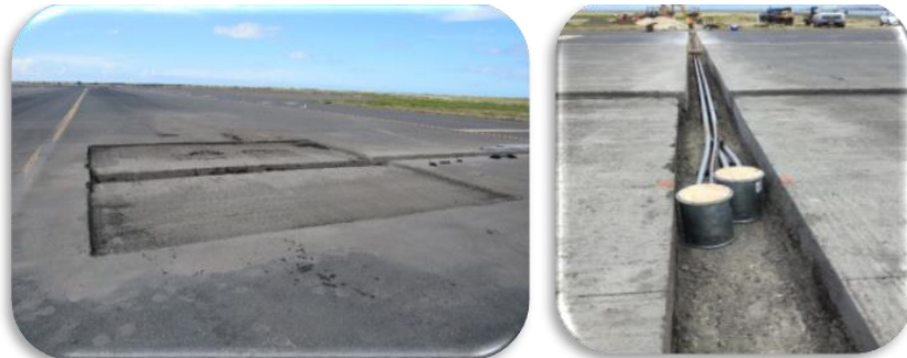
Figure 3. The milled area for the sensor location.
