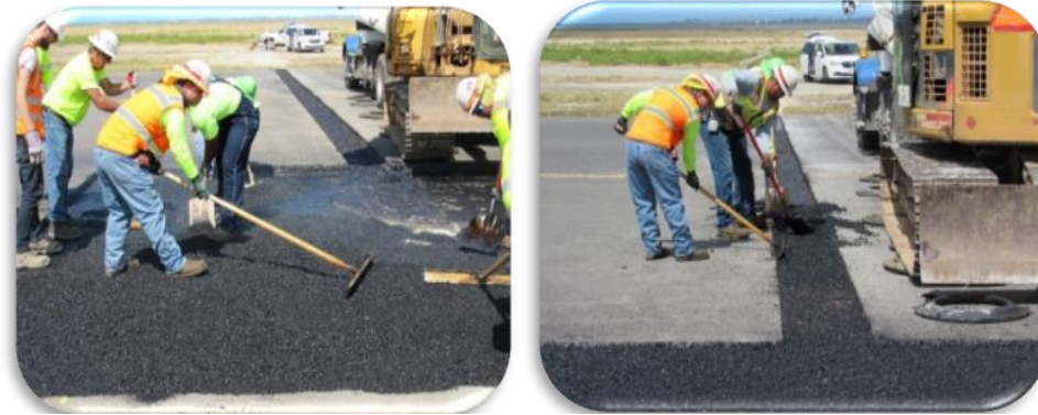
Figure 6. Placing hot mix asphalt.
