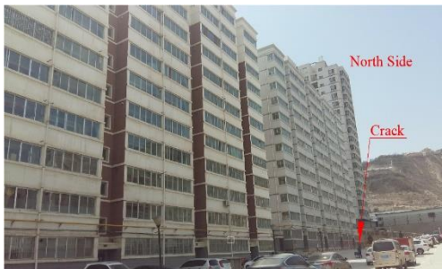
Figure 3. The tilting building.
