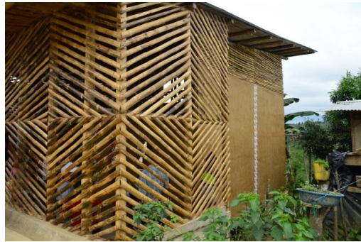
Figure 2. Partially enclosed porch area is semipublic, and the back is private. All-natural materials.
