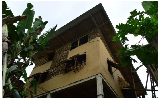
Figure 4. Rear Façade: opens to views.
