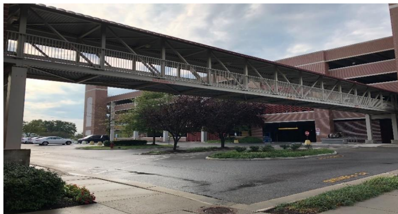
Figure 1. Footbridge used in the study.
