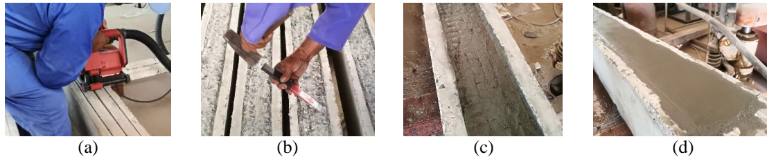
Figure 2. FRCM Strengthening: (a) grooving the beam, (b) chipping the concrete and clearing the groove, (c) applying first layer of mortar and impregnating the fabric, (d) finishing after FRCM application.
