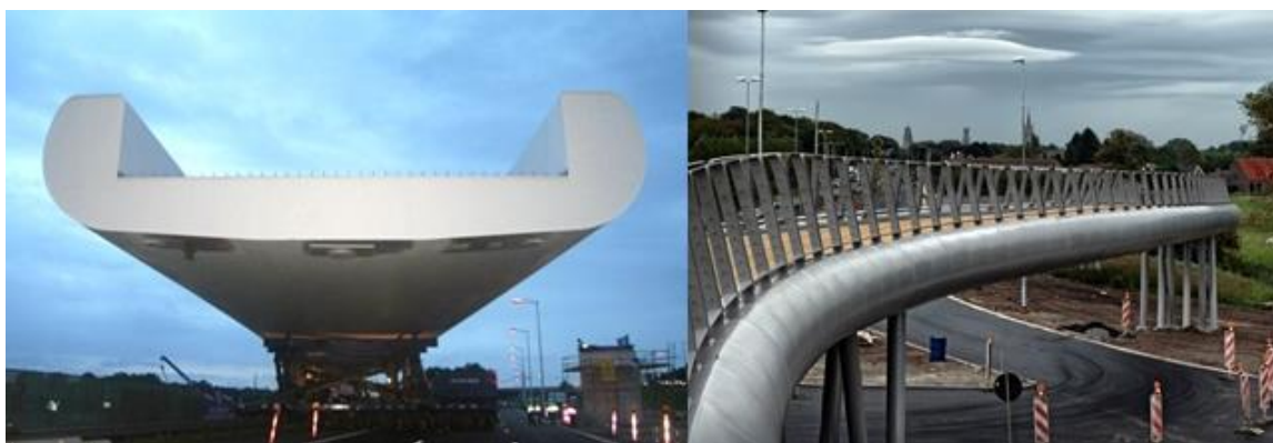
Figure 1. Railway bridge in Zemst and bicycle bridge in Bruges.
