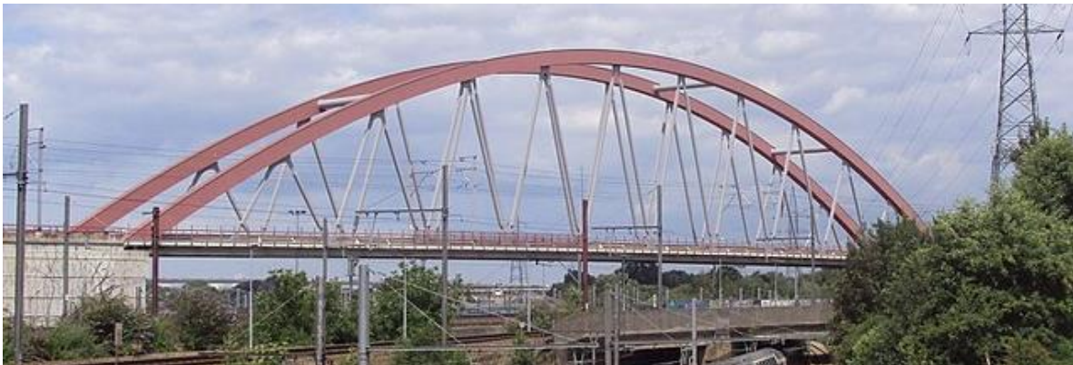
Figure 2. Schaarbeek railway bridge with span of 140 m.
