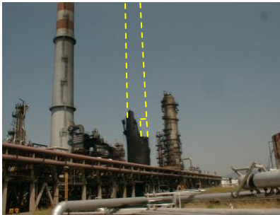
Figure 1. Collapse of Tupras chimney (Photo by P.L. Gould 2004).
