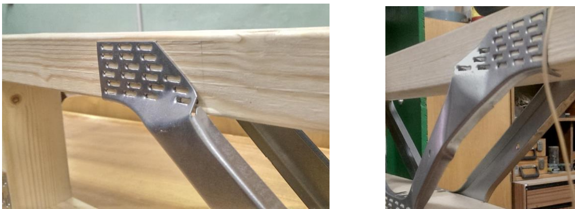
Figure 3. Characteristic failure mode of “Easi-Joist” model.
