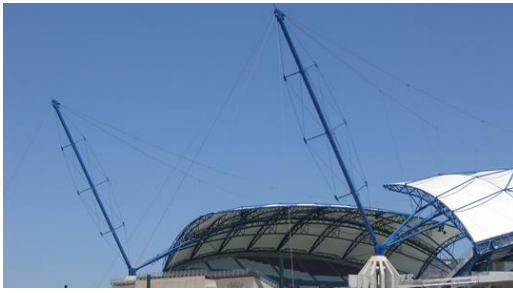
Figure 1. Stadium in Faro (Portugal) with triple crossarms, each with three in-space arms (photo J. Machacek), critical and collapse loads for stayed columns with just one central crossarm.
