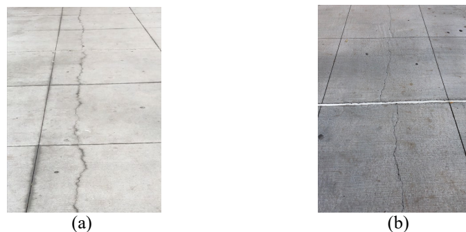
Figure 4 (a), (b). Cracks in sidewalk concrete slabs on Park Ave. in New York City.
