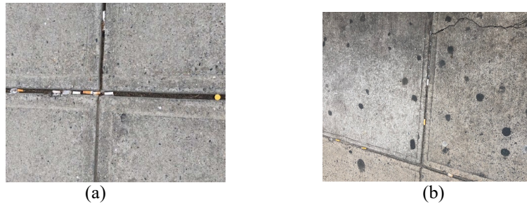
Figure 3 (a), (b). Cigarette ends trapped in saw-cut grooves in walkway slabs.
