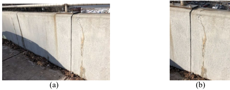
Figure 6 (a), (b). Cracks in NY bridge parapet walls with saw-cut joints.
