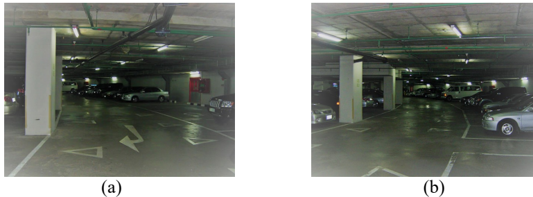
Figure 9. Crack-free garage basement floor in UN-ESCAP Conference Building (Seniwongse 1991).
