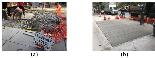
Figure 8. (a) Removal of cracked walkway slab, (b) Recast walkway slab.
