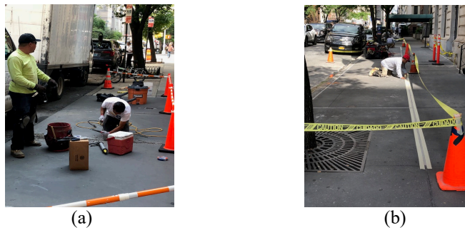
Figure 7. (a) Saw cutting grooves in walkway slab, (b) Taping saw-cut groove before applying sealant.
